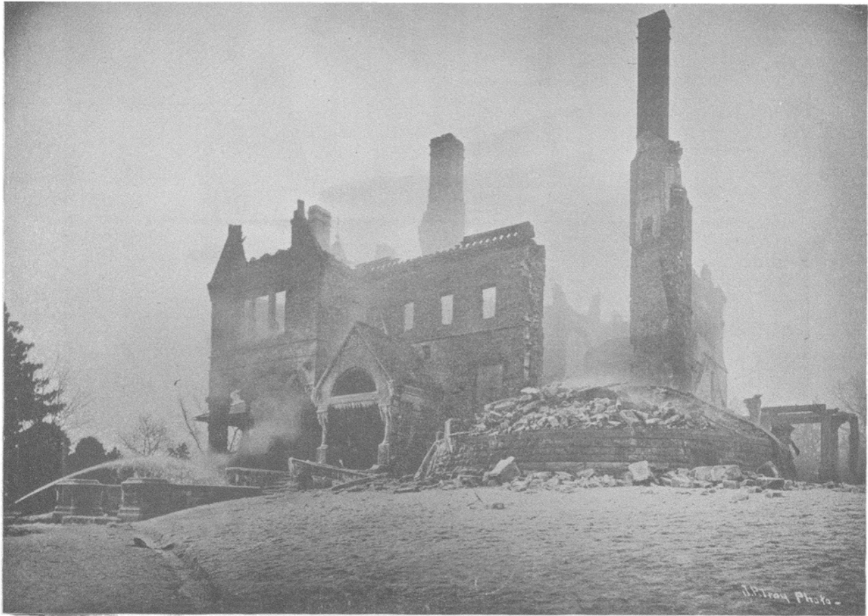
RUINS OF THE CHI PSI HOUSE JUST AFTER THE FIRE.
